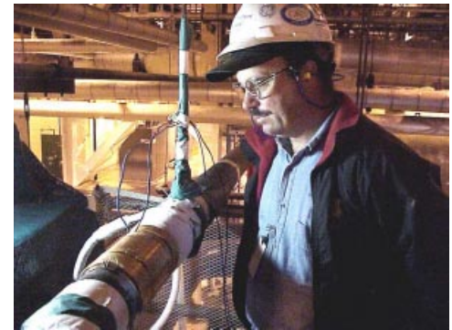
Dennis Schrempp inspects the piping upstream of FP-V-230.
